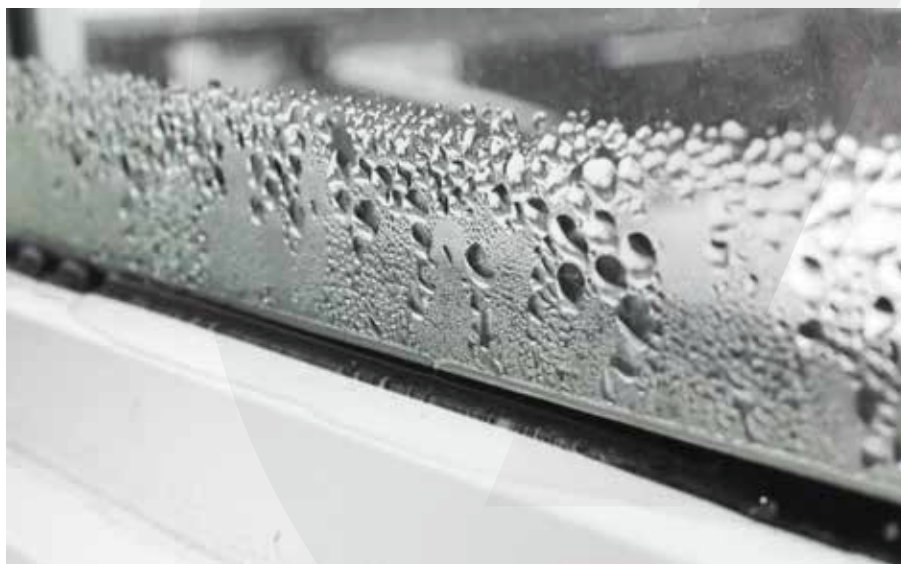
Fig. 25 Moisture condensation on external glass pane of the insulating glass unit.
