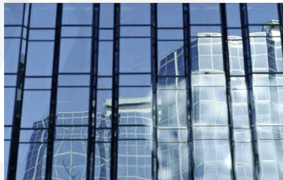
Fig. 24 Distortion effect, depending on concavity/convexity of glass panes due to overall bow and roller wave of toughened glasses, etc.
