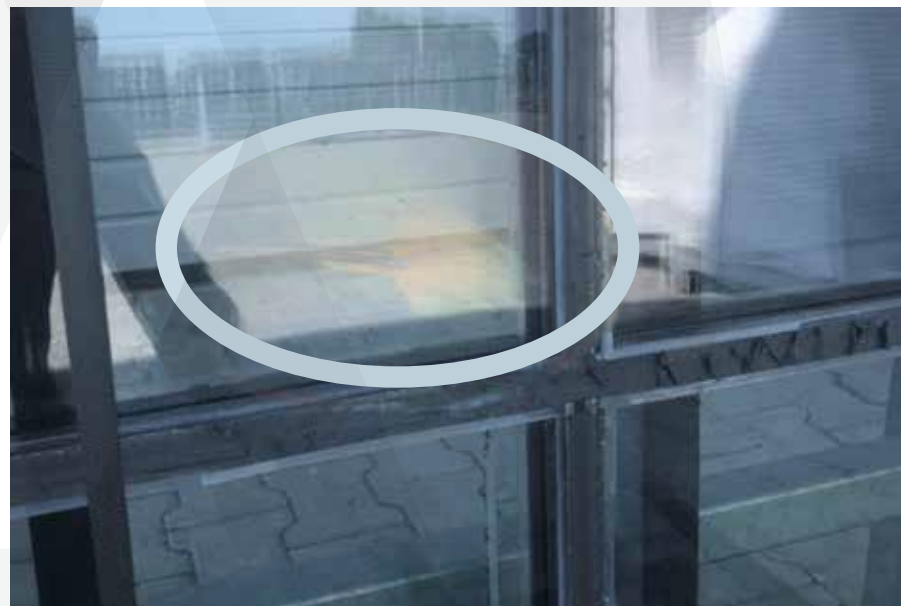
Fig. 29 Chemical evaporation inside the insulating glass unit after exceeding recommended temperature of 60 °C
