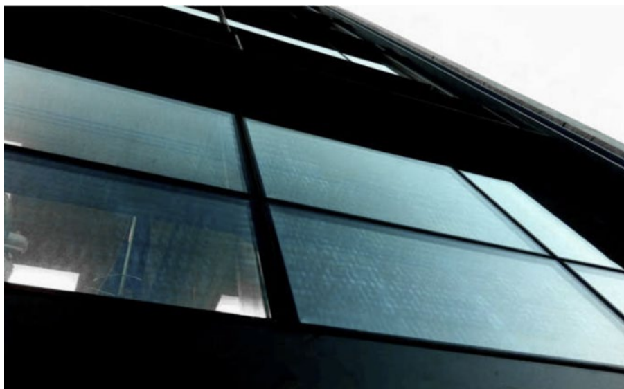
Fig. 27 Anisotropy in heat-treated glass
